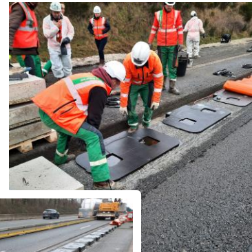
Coils laying & gluing
