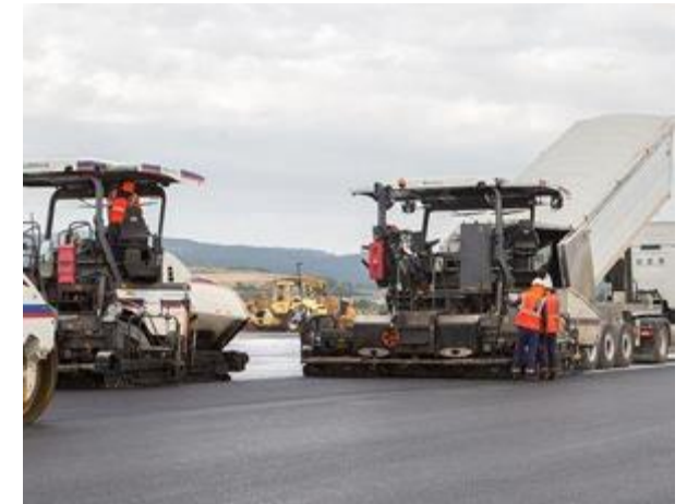
200m surface course repair test
