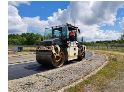
Asphalt and compaction
