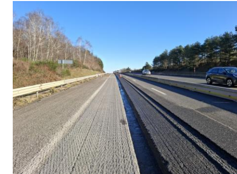
Road milling & trenches
